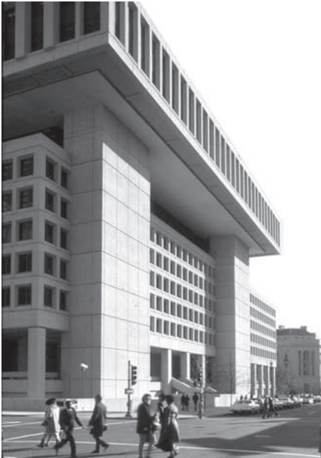
J. Edgar Hoover F.B.I. Building, Washington, DC Photo credit: Dr. Richard W. Longstreth
