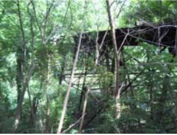
The Foundry Branch Trolley Trestle. DCPL Archives.
