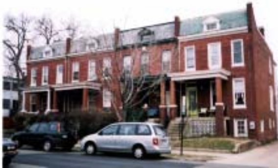
Top: 827-833 Kentucky Avenue SE. Bottom: 712-718 16th Street SE. DCPL Archives.
