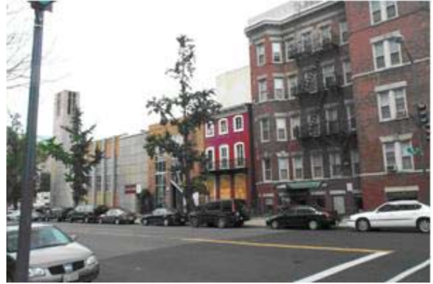
Judiciary Square Clusters: The 300 block of E Street exemplifies the few remaining clusters of buildings from the mid nineteenth and early twentieth centuries. (DCPL Archives)
