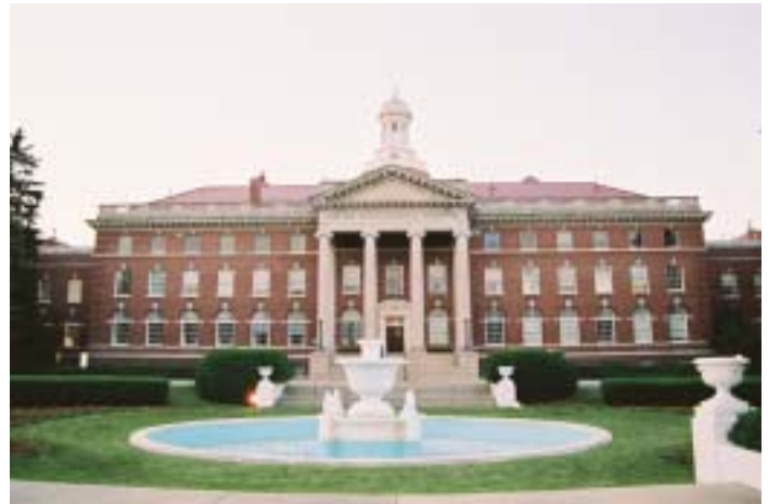
Walter Reed, 6900 Georgia Avenue NW: Pictured is the main hospital building. (DCPL Archives)
