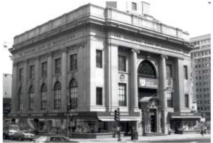
Above: The Federal-American National Bank (the future home of the Armenian Genocide Museum of America), built in 1925-26, was designed by nationally prominent bank and skyscraper architect Alfred C. Bossom in association with distinguished Washington architect Jules Henri De Sibour, the city's leading practitioner of the Beaux-Arts style. The building's design incorporates a number of innovative interior and exterior features, most notably the elevated two-story banking hall, which is one of only twelve landmarked interiors in the city.
